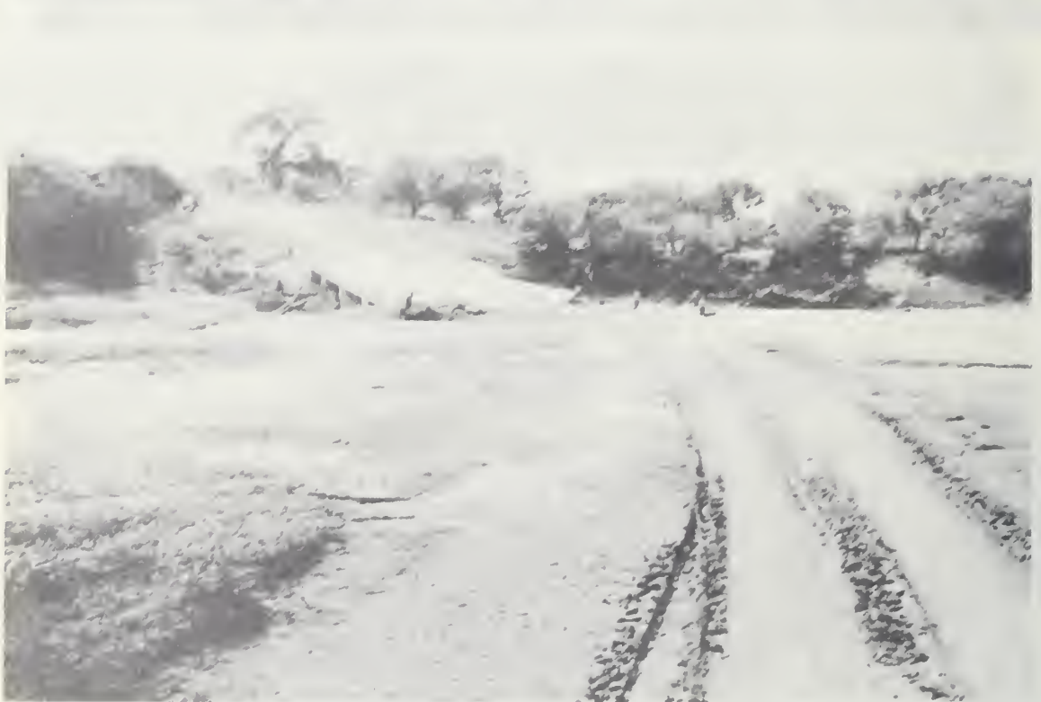
Average annual damages to roads and bridges exceed $2,700.
